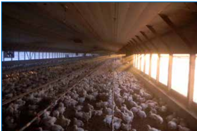
Figure 28: An example of natural ventilation.
