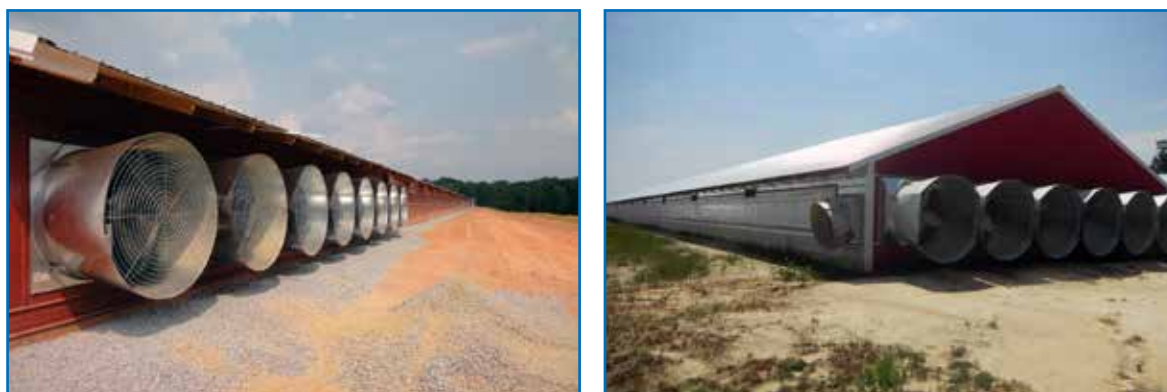
Figure 40: Example of a typical tunnel ventilated house.
